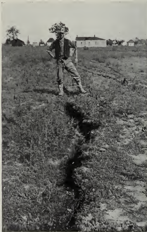
FIG. 6.—Crack in the soil, caused by room-and-pillar mining at a shallow depth at Streator.
